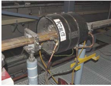
Figure 1: The HERA-e DCCT installation: a simple construction with water cooling.
