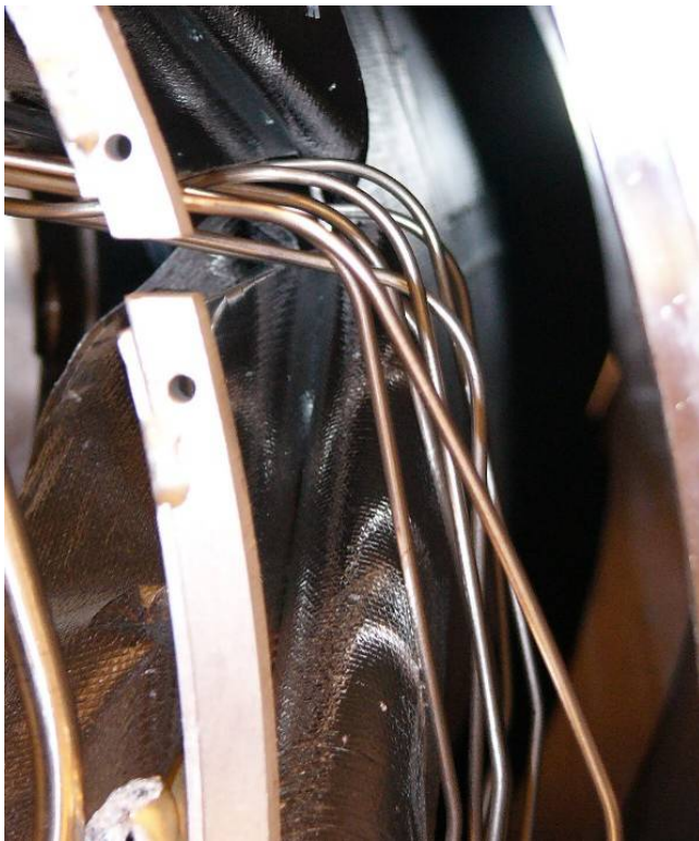
Forming was not found to be as accurate as was specified.
